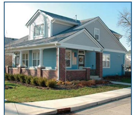
The Millennium Place HOPE VI redevelopment includes rental housing for seniors and families, and market-rate and low-income homes.
